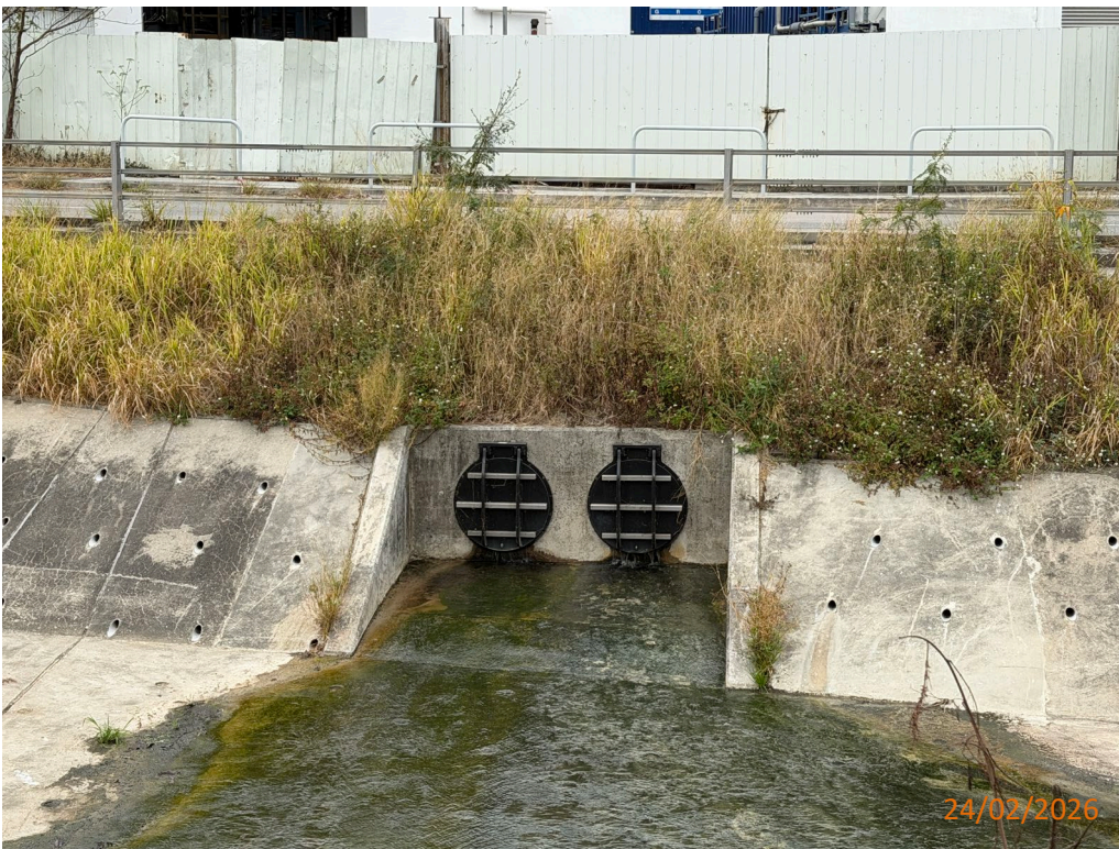
Existing drainage facilities
